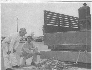
MAGNET MAGIC is pointed out to Alfredo Fernandez, left, by Carlos M. Ortega who shows the results of a trip through the Tech Area and parking lots in a truck carrying an electro-magnet. The generator in the back of the truck powers an amazingly strong electro-magnet slung near the ground behind the truck. Here the big girder-like magnet is shown with the pile of metal scrap drawn up from the tech area streets and the parking lots. This cleanup is made by men from 2417 about every six weeks.
